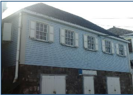
Pic D - The Post Office, refurbished in 2004. Located in the center of Charlestown, adjacent to the Nevis Tourism Authority building.
