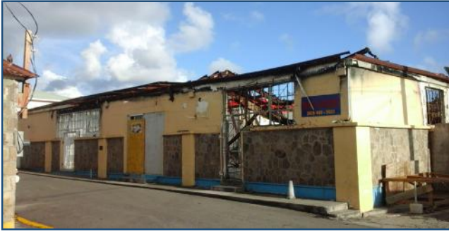
Pic C – The treasury building recently joined the list of abandoned buildings after destroyed by fire in 2014.
