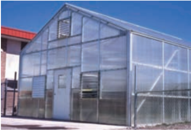
Figure 1.11 —Good site assessment and an understanding of your crop’s needs will help you determine the best structures for your nursery. Shown here is the greenhouse at the Browning High School on the Blackfeet Reservation in Montana. Photo by Tara Luna.
