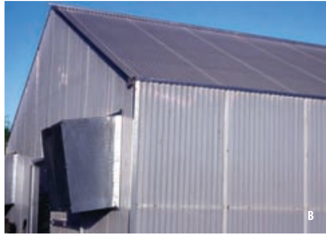
Figure 4.10 —(A) Greenhouses are covered with transparent coverings such as plastic sheeting or (B) hard plastic panels to maximize the amount of sunlight reaching the crop. Photo A by Tara Luna, B by Thomas D. Landis.
