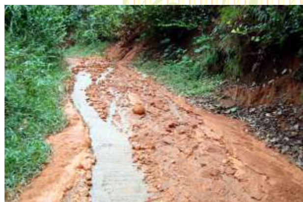
Effect of surface run-off in the upland region
