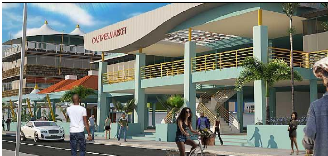
Figure 6: Redevelopment of the Castries Market
