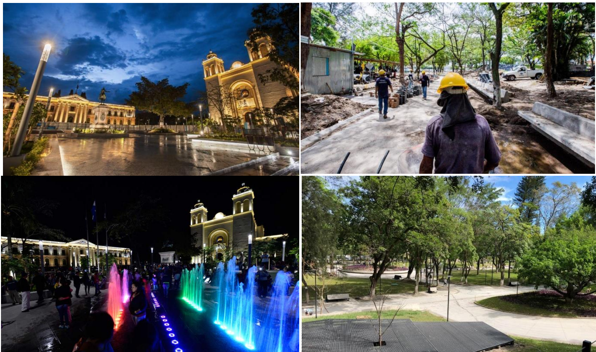
Figure 3: Finished work of Gerardo Barrios Square and progress of works at Cuscatlan Park, phase 1. (Source: City Hall of El Salvador and Prisma Ingenieros)
