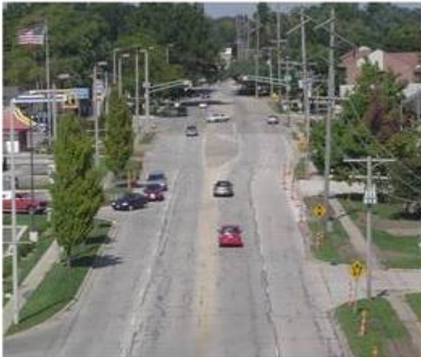
Original four-lane arterial designed to maximize motor vehicle traffic speeds.
