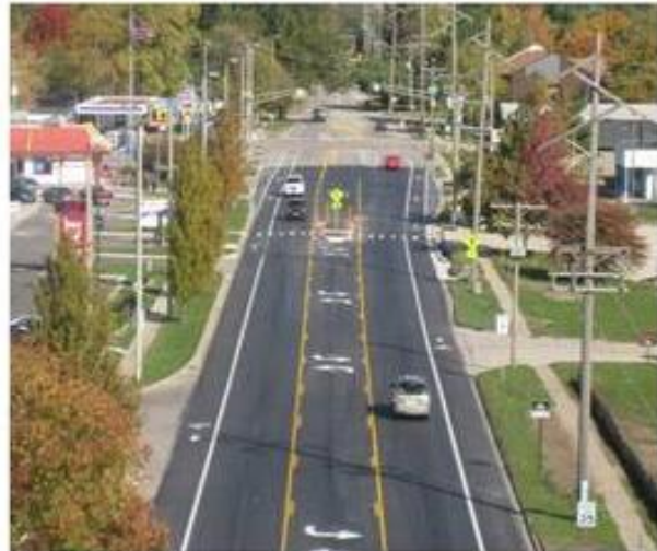
Complete street with center turn lane, bike lane and pedestrian refuge island at bus stop.
