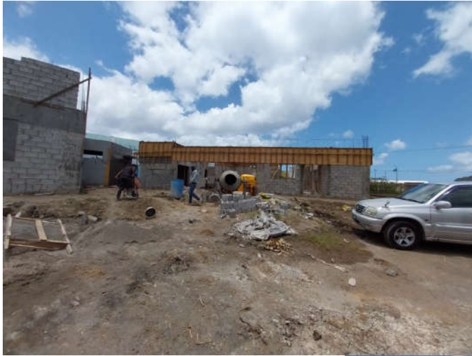
Walls & Rim beams
